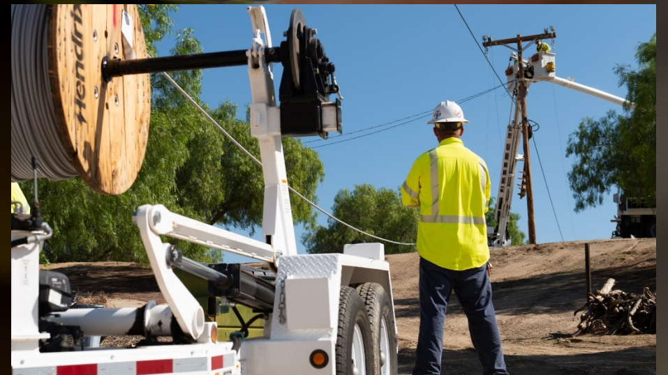
Above photos: SCE crew installing insulated wire
